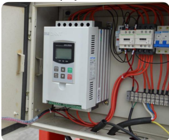
Soft Start to protect electric motor
