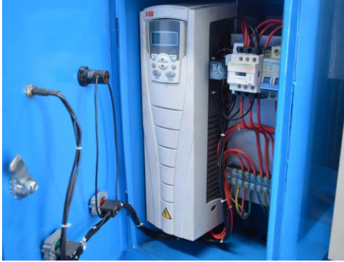
LH65 squeeze hose pump drive (ABB)
