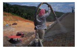
LZ-3A Air motor dry mix concrete spraying machines small-sized shotcrete machine for the dry spraying process. LZ-3A dry mix concrete spraying machine can be used as well for small jobs, such as joint filling, swimming pool, refractory application and extensive slope consolidation work, etc.
